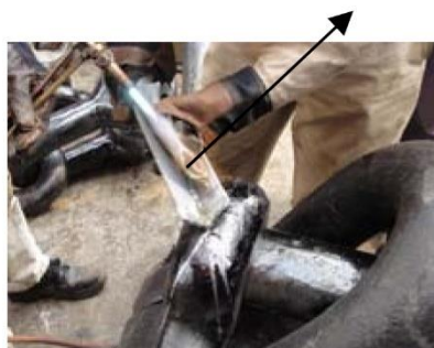
heating the lead and fill-up
