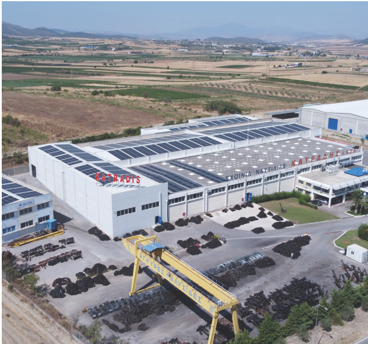
Katradis AVEE after the installation of the photovoltaic system.
